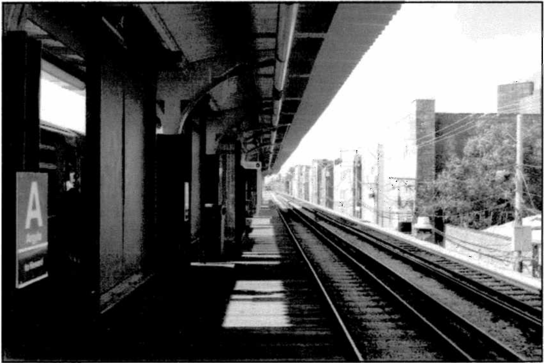
West Argyle Street elevated platform (1922)
